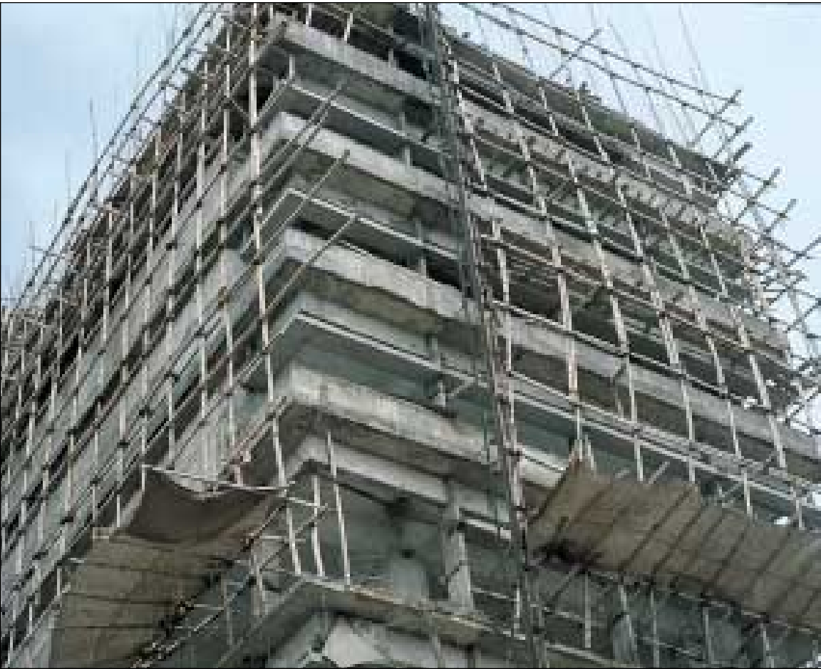
Fig. 7. Bamboo scaffolding, mainly from Bambusa balcooa and B. vulgaris , Dhaka, Bangladesh.
